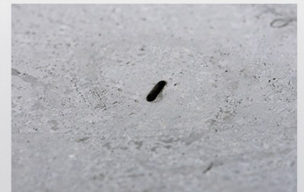
Low pressure piercing - ON
